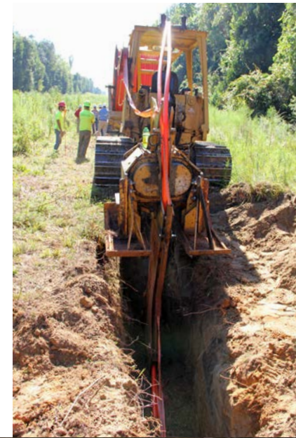
Georgia Transmission crews prepare a trench for fiber optic cable installation.
