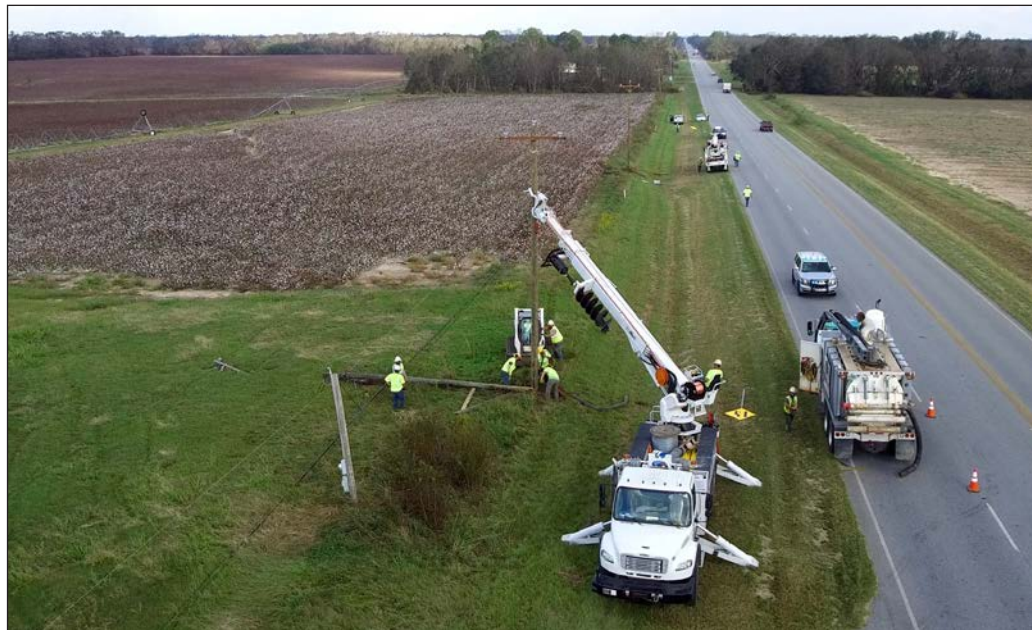
Below: Crews repair a transmission line in Southwest Georgia.
