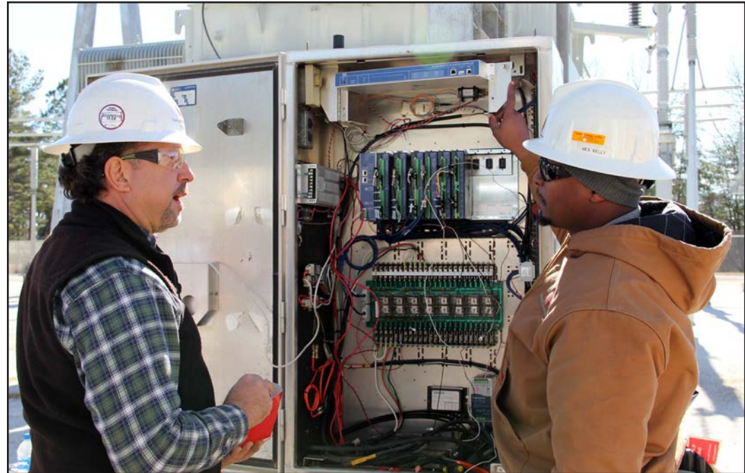
Georgia Transmission employees test updated substation communications equipment.
