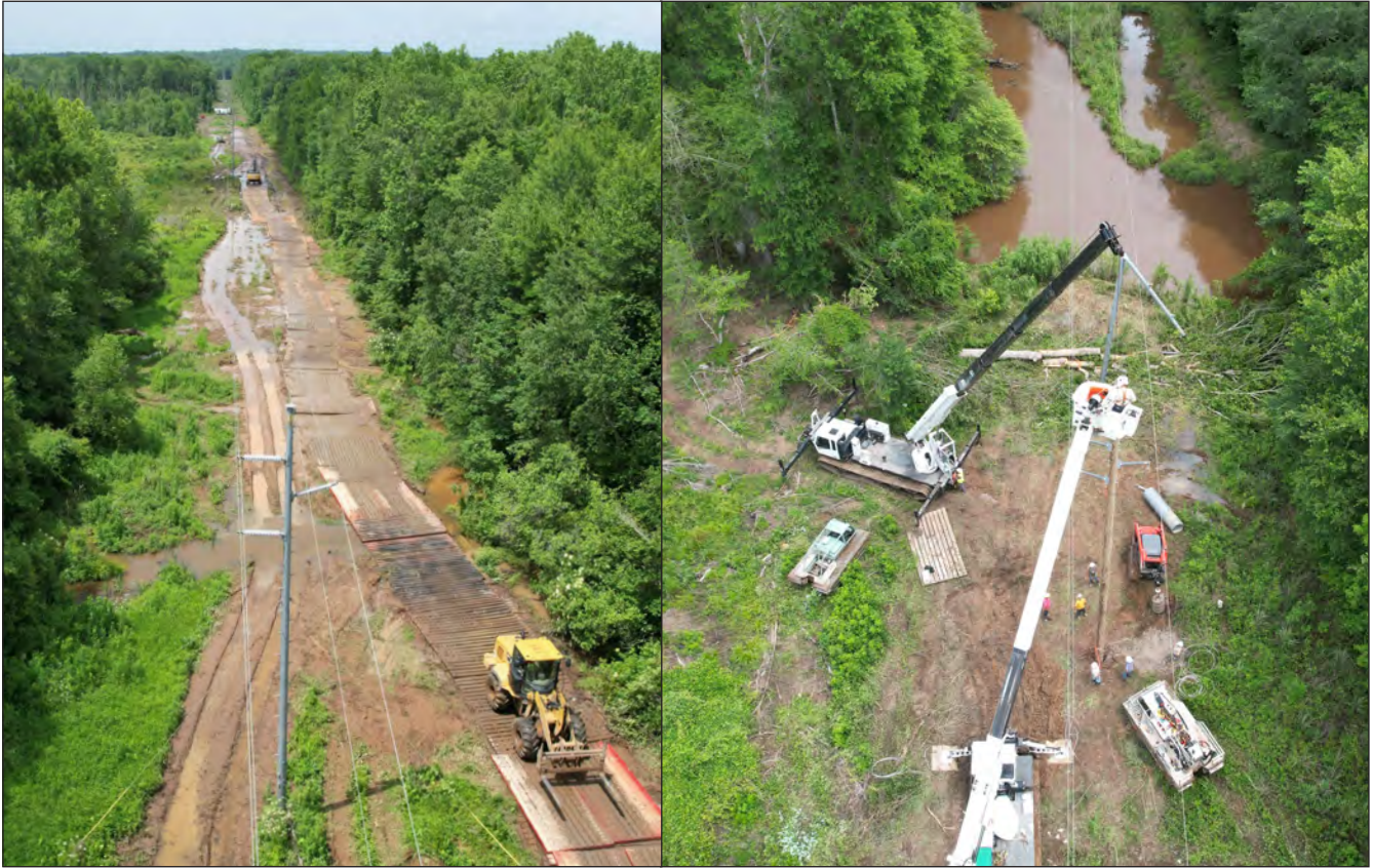
To meet the challenge of reaching a downed line in a rural area, Georgia Transmission used more than 800 wooden mats, spanning more than a mile, across swampy terrain to move the necessary equipment to the damage site.
