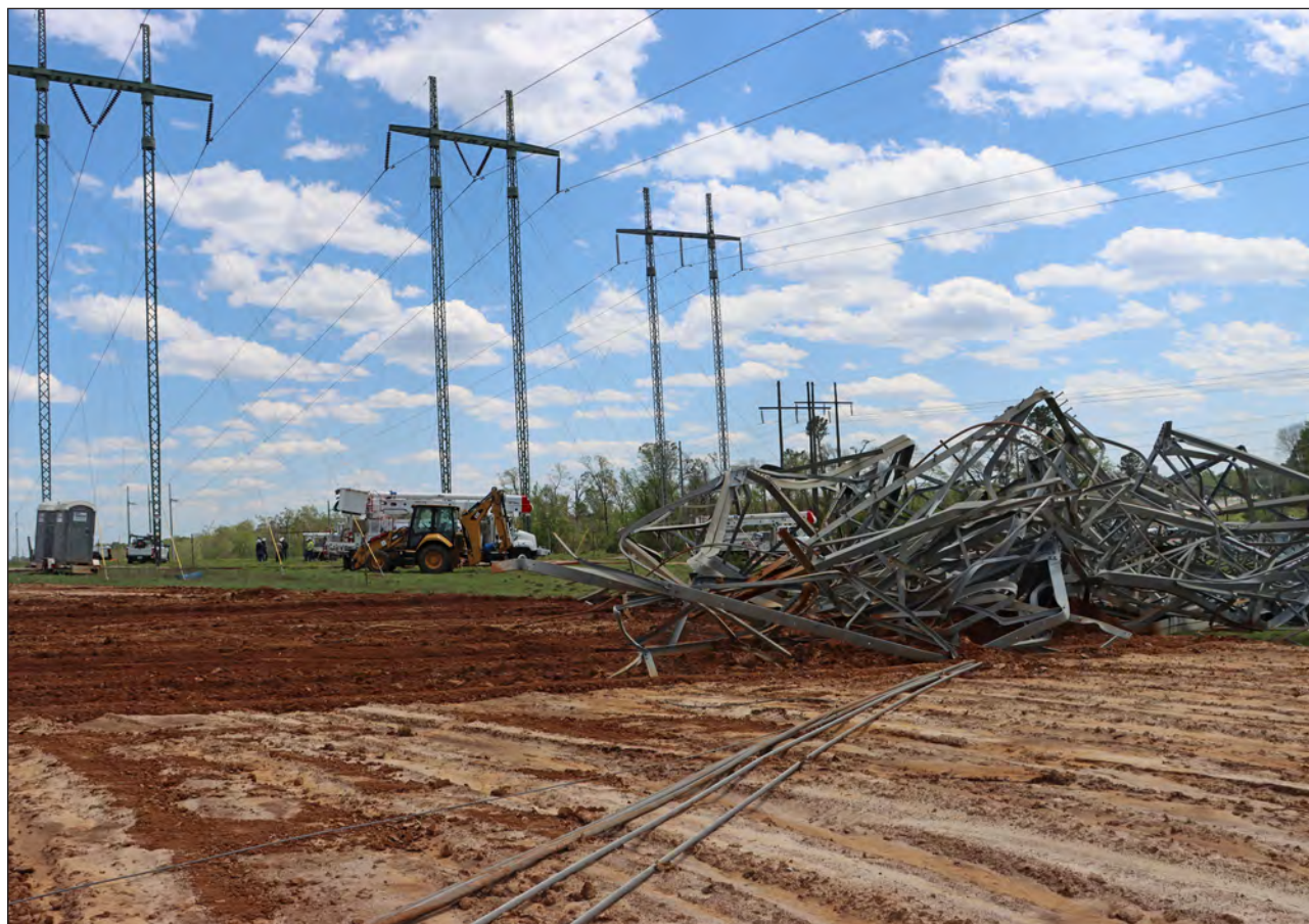
After a tornado took down two 500 kV towers near Bonaire, Georgia, we quickly restored power as a result of our grid-resiliency investments. Through long-standing partnerships and agreements with members of Georgia's Integrated Transmission System, we rebuilt the towers within three weeks.
