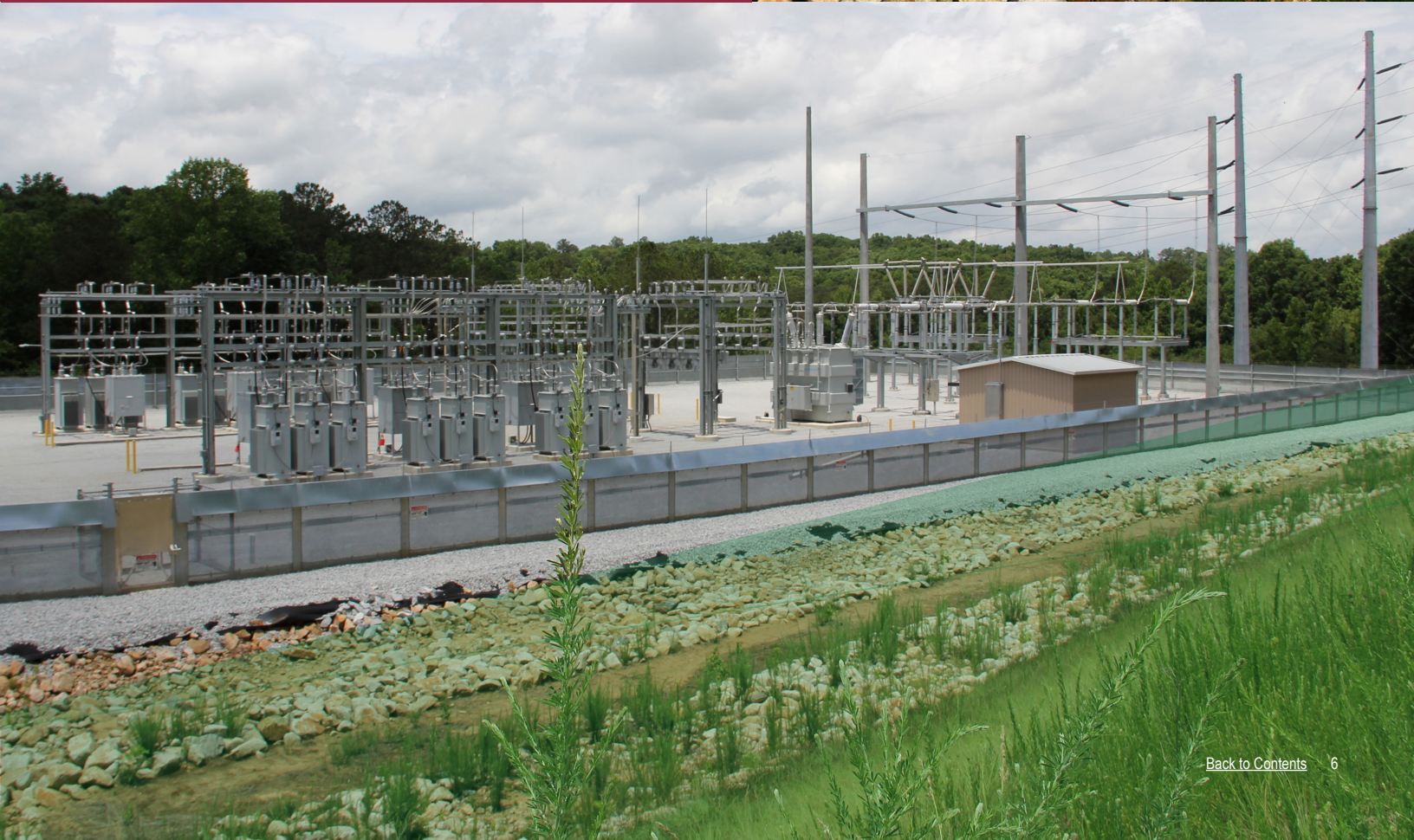
For the Wolf Creek Substation, a plateau was constructed to provide a stable foundation with a front wall soaring to a height of more than 50 feet.
